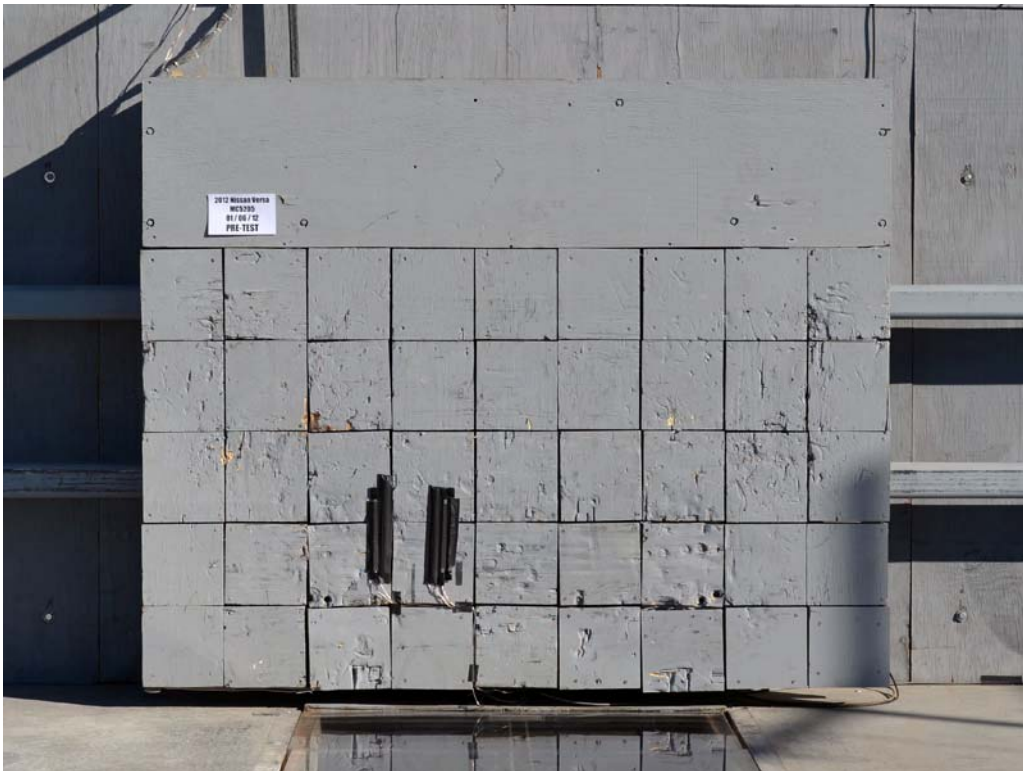
FIGURE 2. Load Cell Wall
