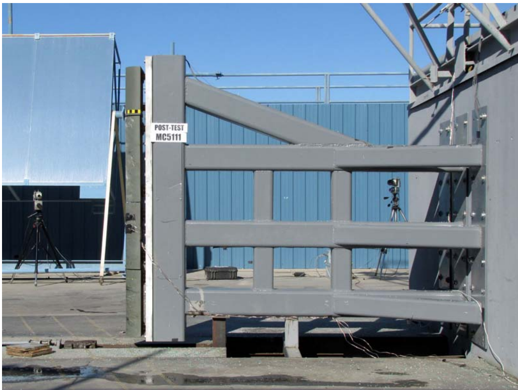
FIGURE 59. Post-Test Pole Barrier Side View
