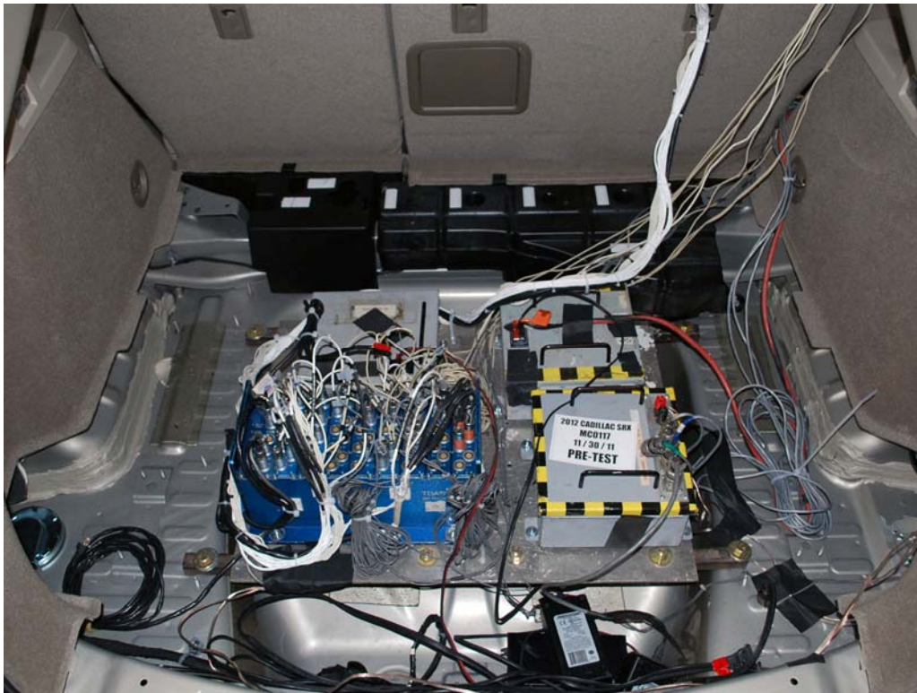
FIGURE 60. Pre-Test Ballast View
