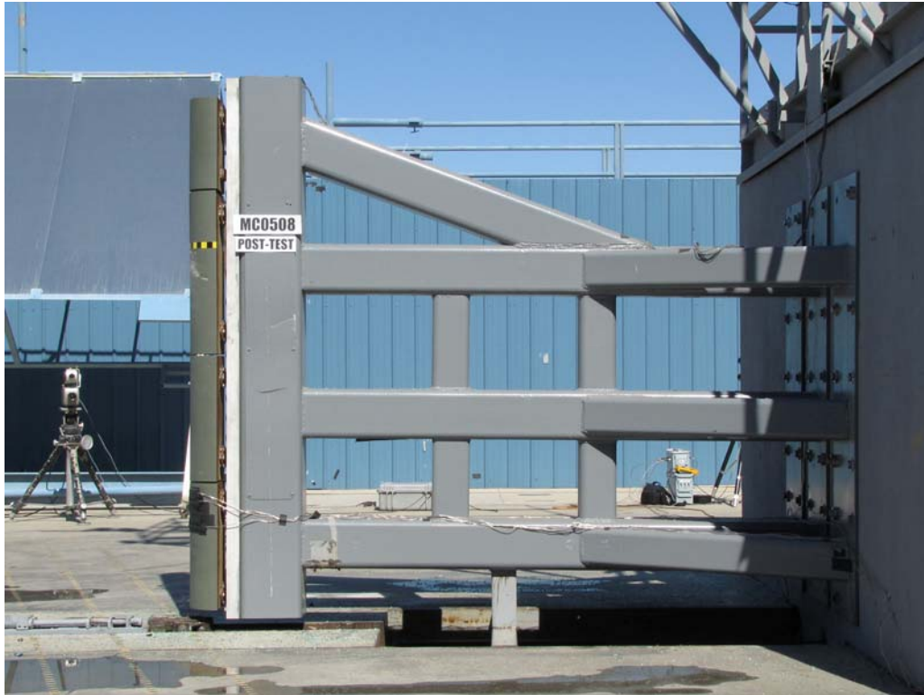
FIGURE 59. Post-Test Pole Barrier Side View
