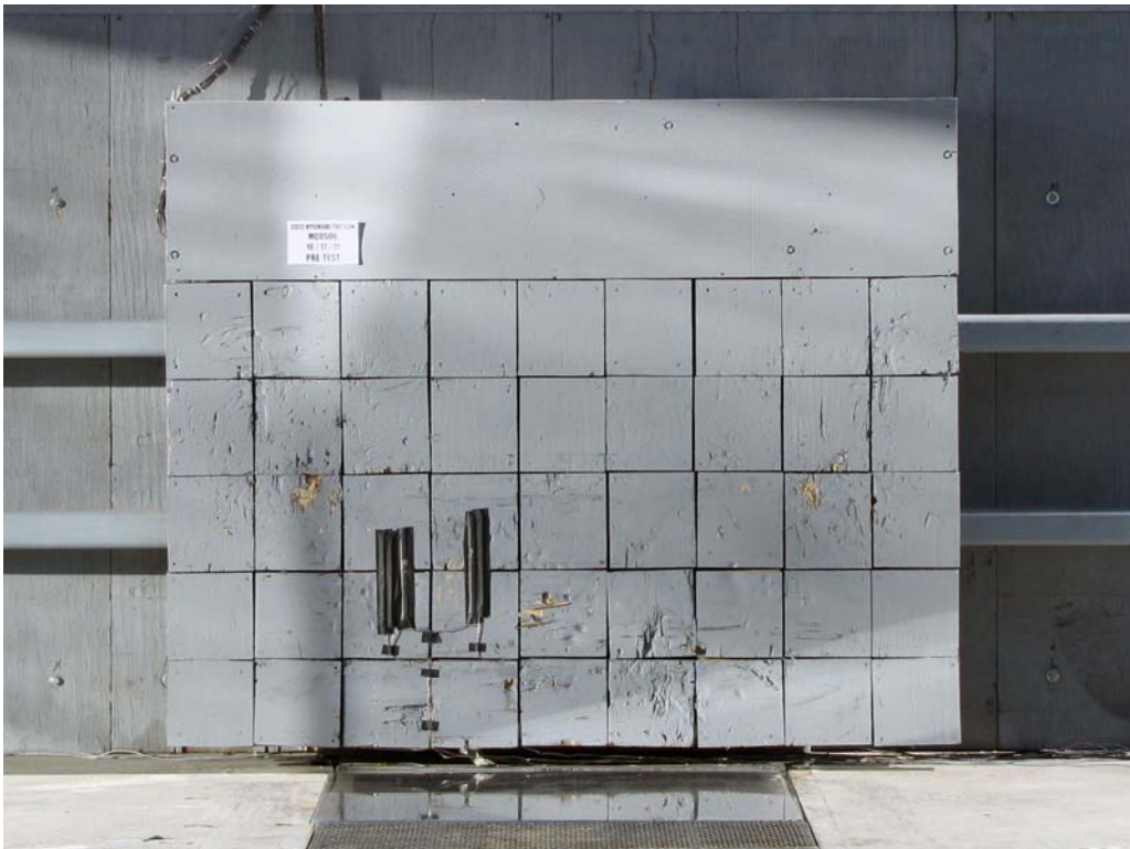
FIGURE 2. Load Cell Wall
