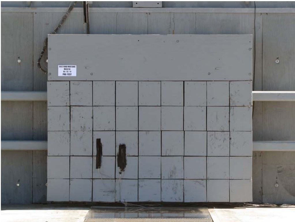
FIGURE 2. Load Cell Wall
