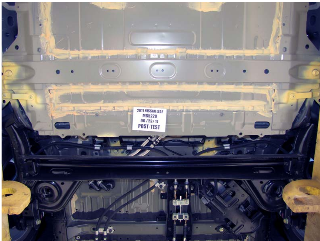
FIGURE 91. Post-Test Battery Mounting Hardware
