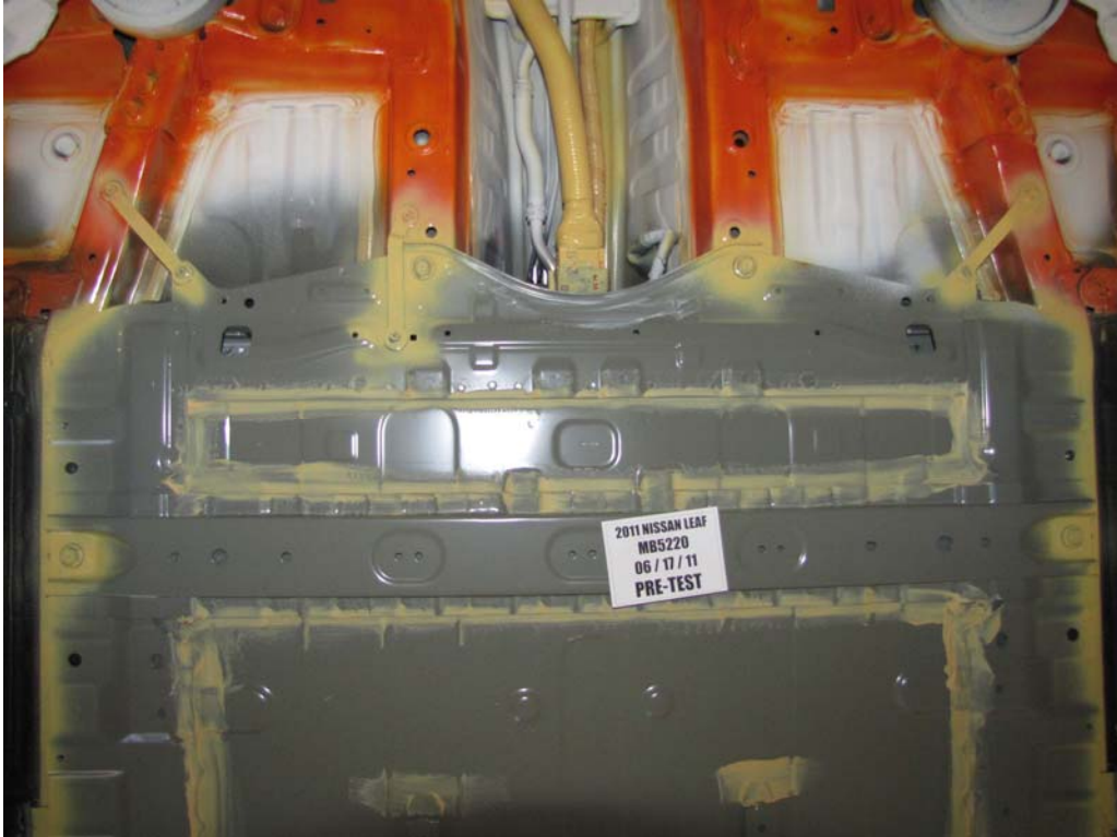
FIGURE 84. Pre-Test Battery Mounting Hardware
