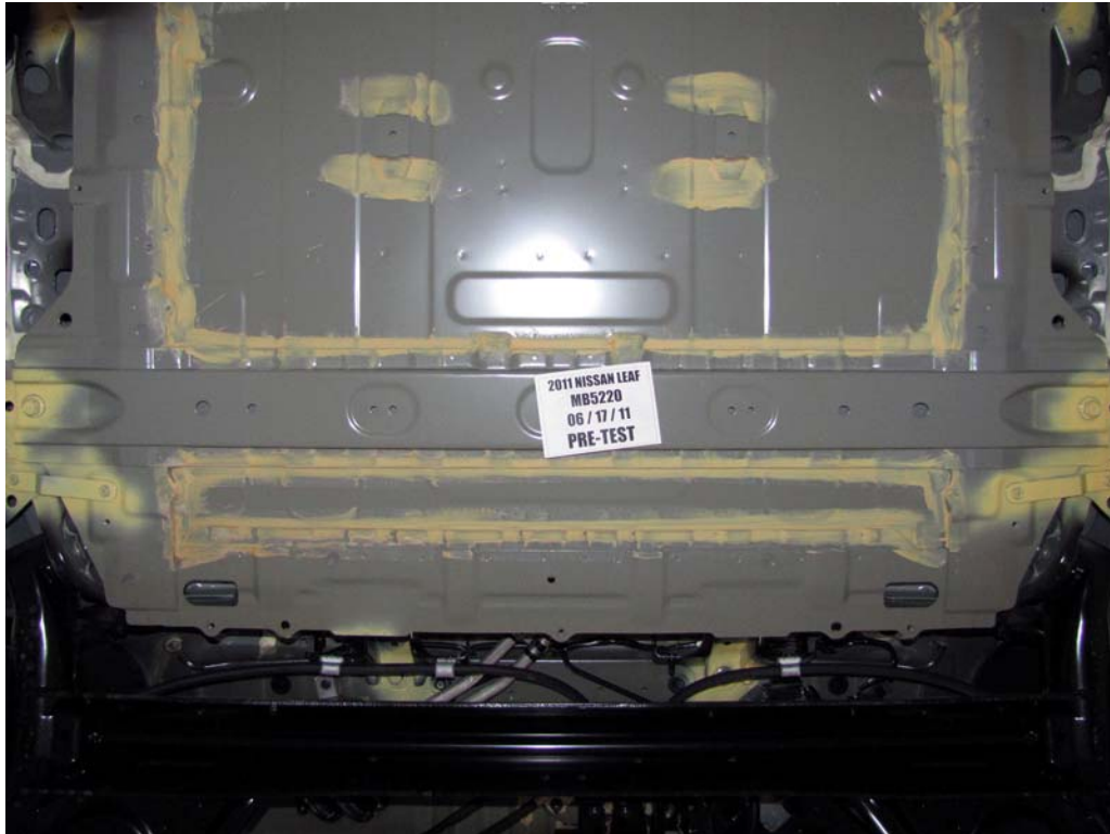
FIGURE 90. Pre-Test Battery Mounting Hardware
