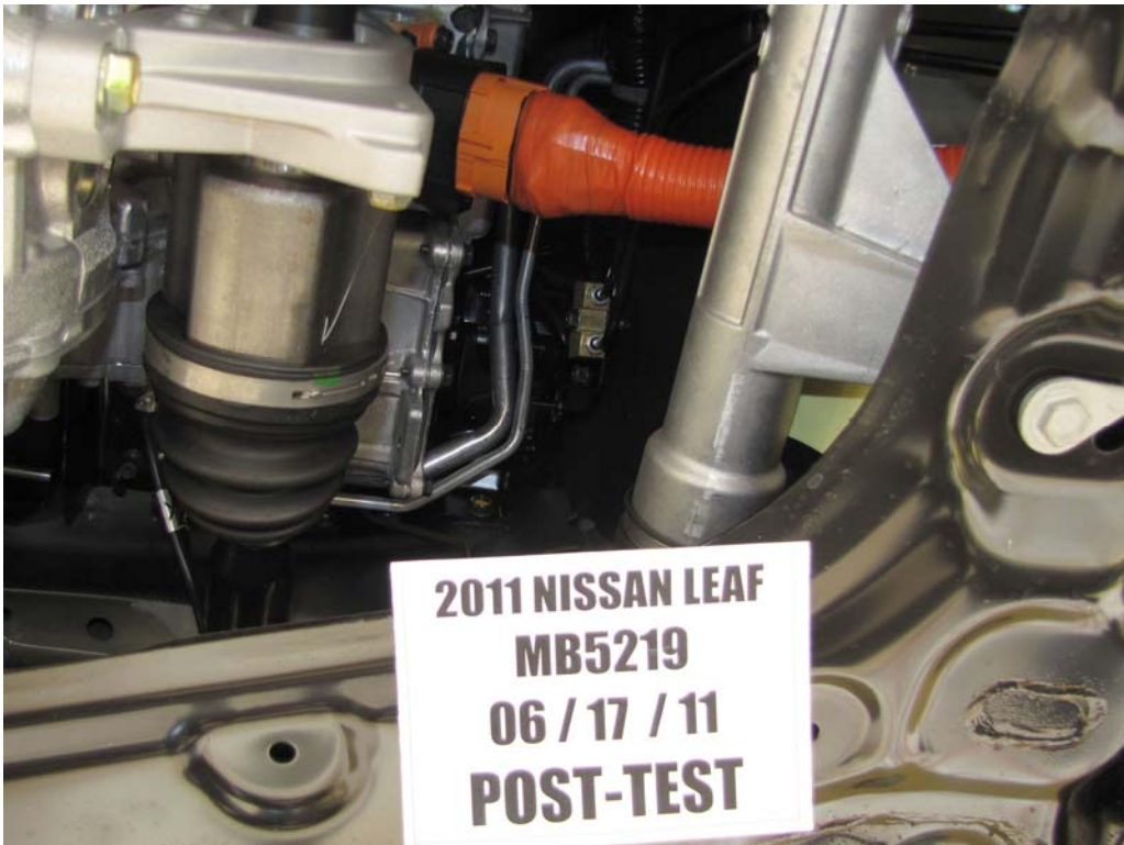
FIGURE 132. Post-Test High Voltage Connections
