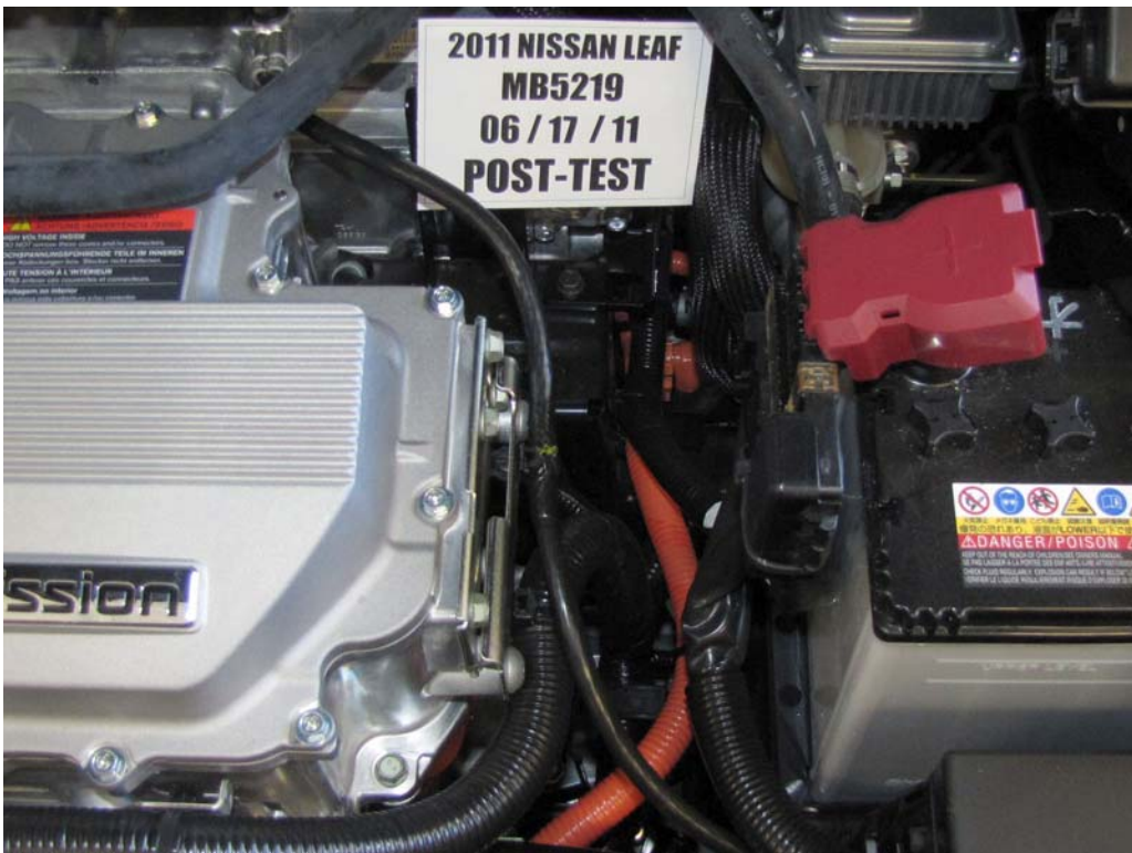
FIGURE 126. Post-Test High Voltage Connections
