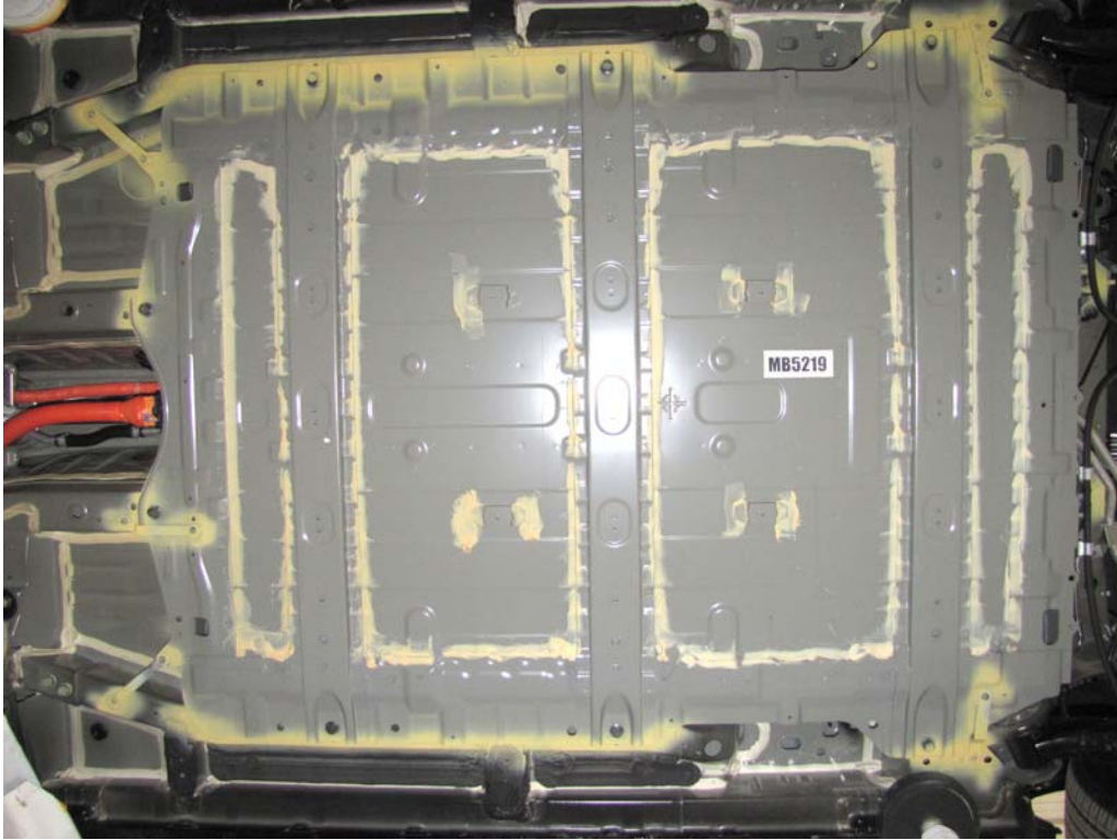
FIGURE 113. Pre-Test Battery Pack Assembly
