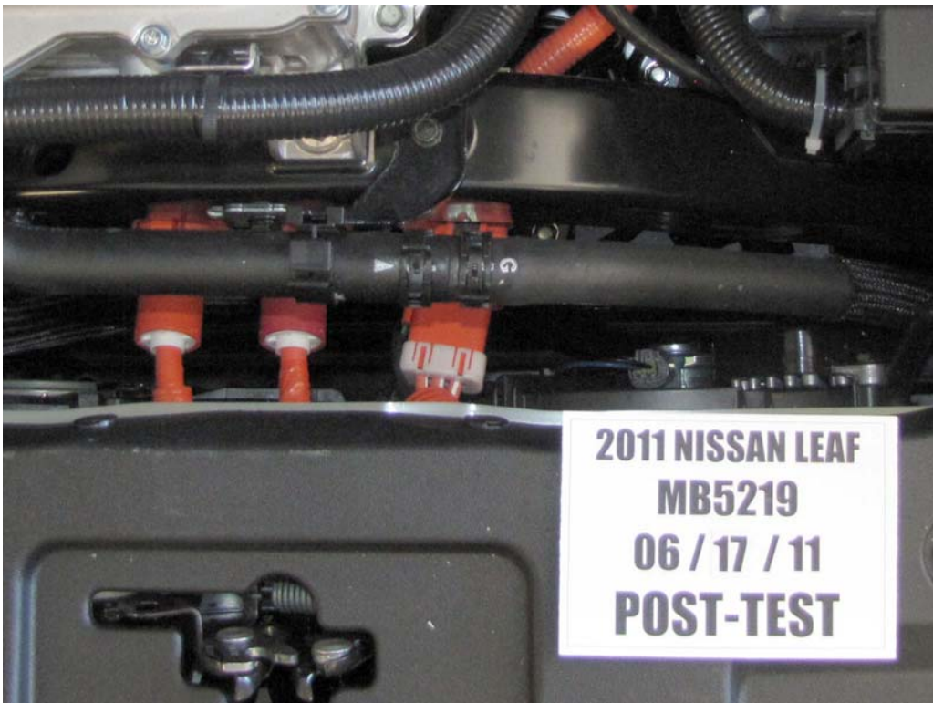
FIGURE 124. Post-Test High Voltage Connections
