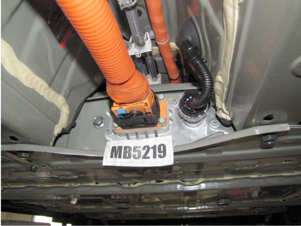
FIGURE 133. Pre-Test High Voltage Connections
