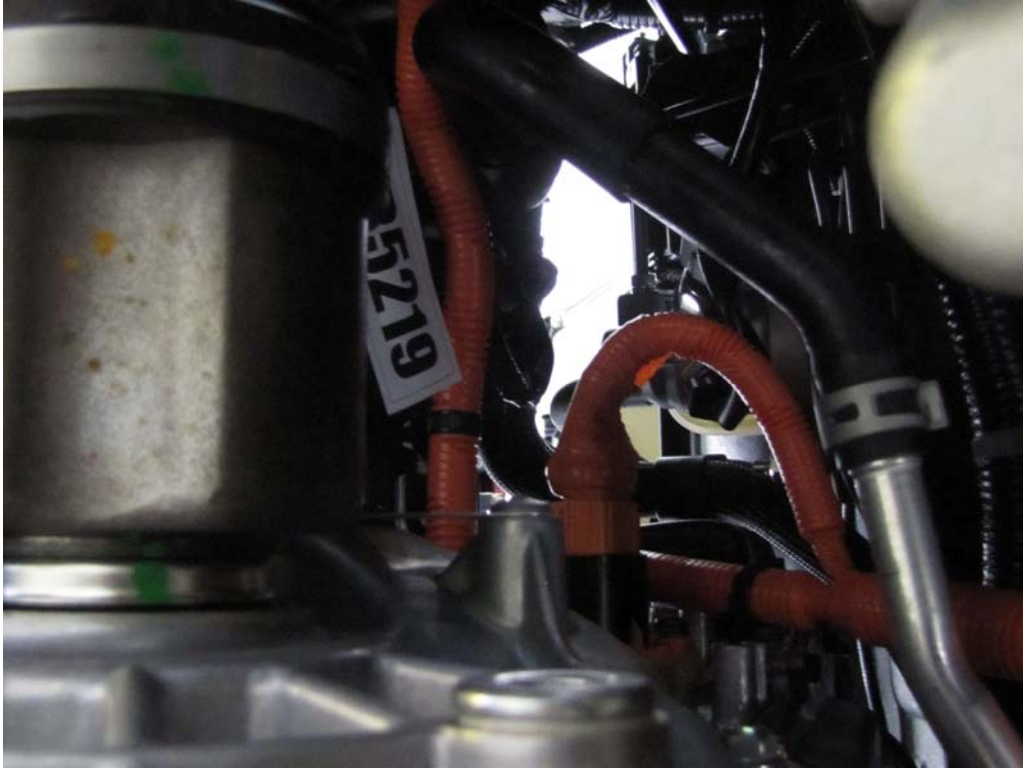
FIGURE 129. Pre-Test High Voltage Connections
