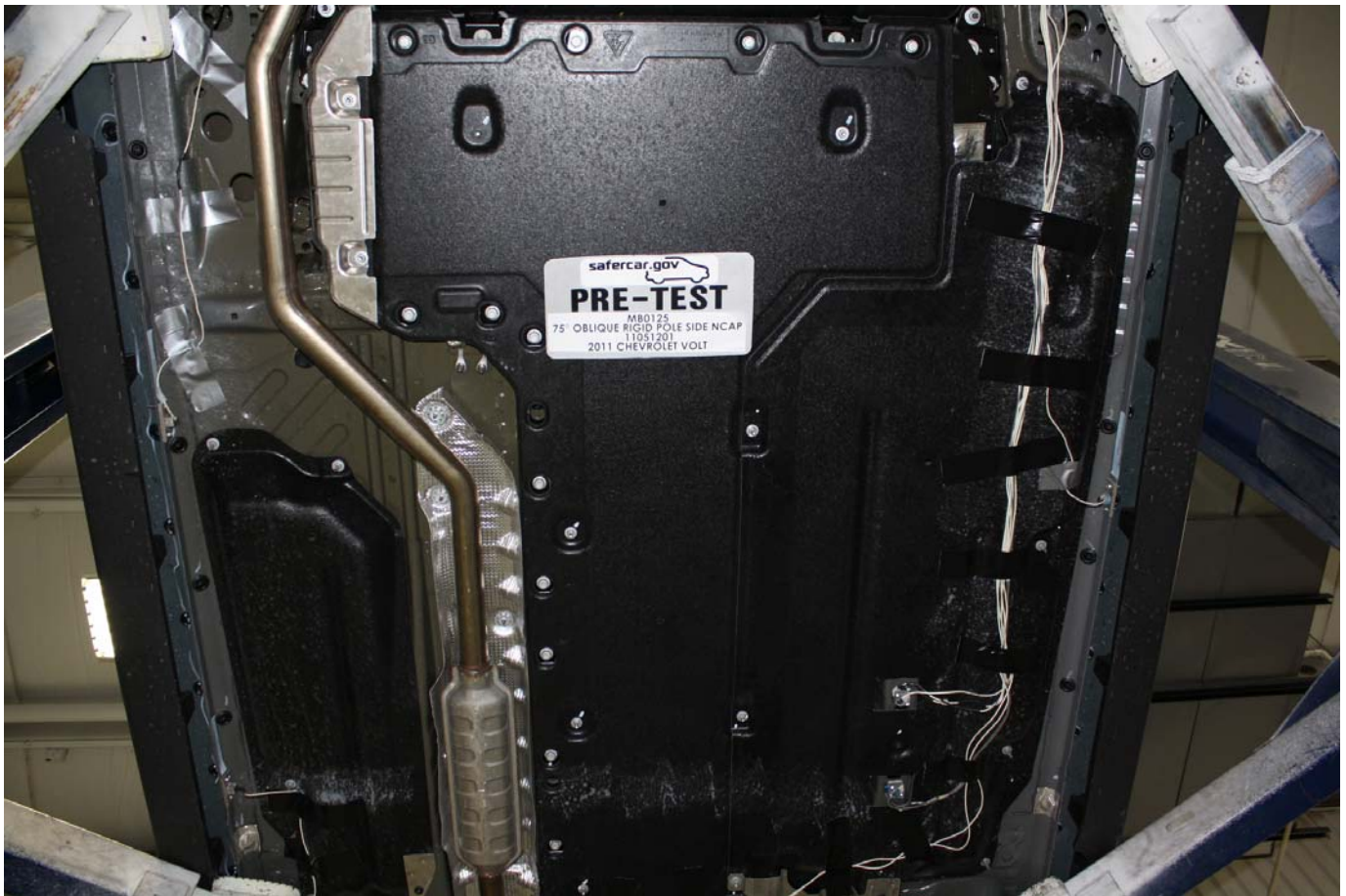
Pre-Test View of Propulsion Battery
