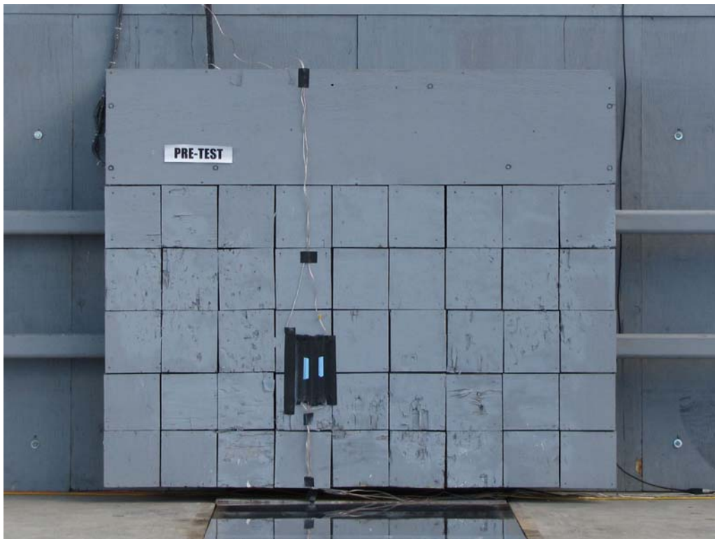
FIGURE 2. Load Cell Wall
