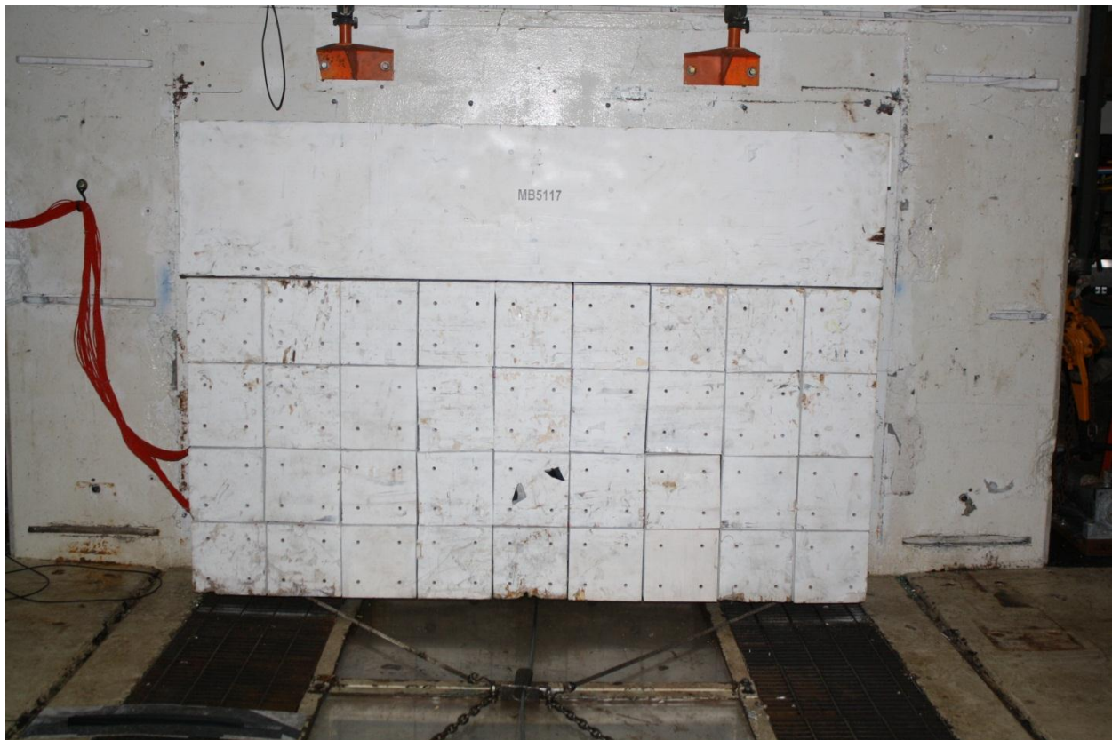
Figure A-2: Load Cell Wall
