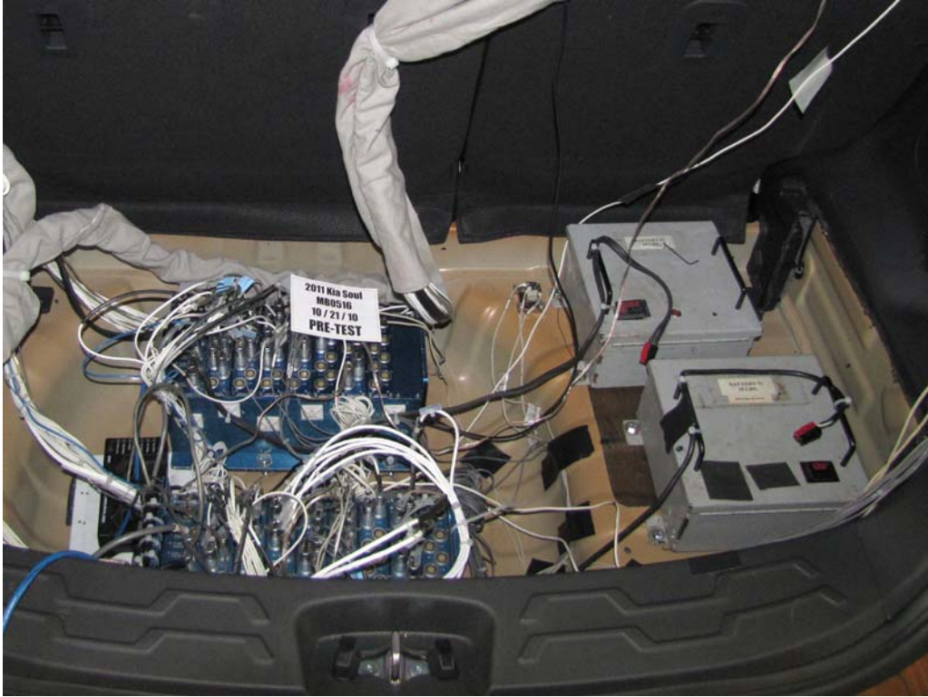
FIGURE 91. Pre-Test Ballast View
