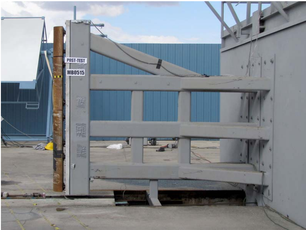
FIGURE 58. Post-Test Pole Barrier Side View
