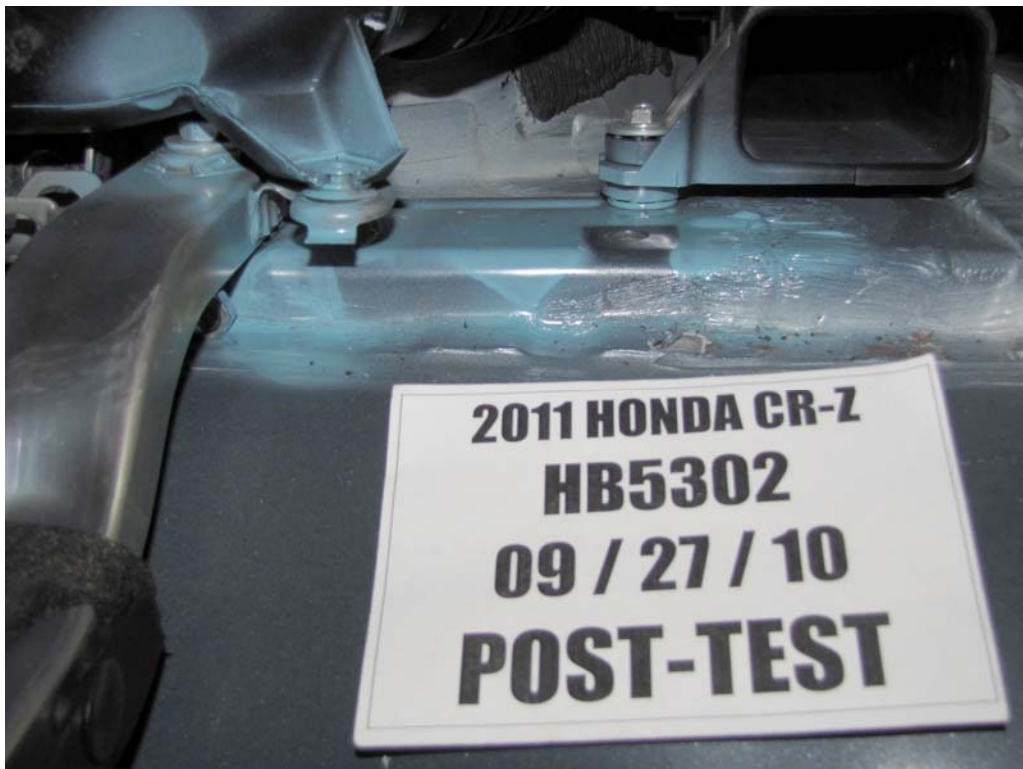
FIGURE 98. Post-Test Battery Mounting Hardware
