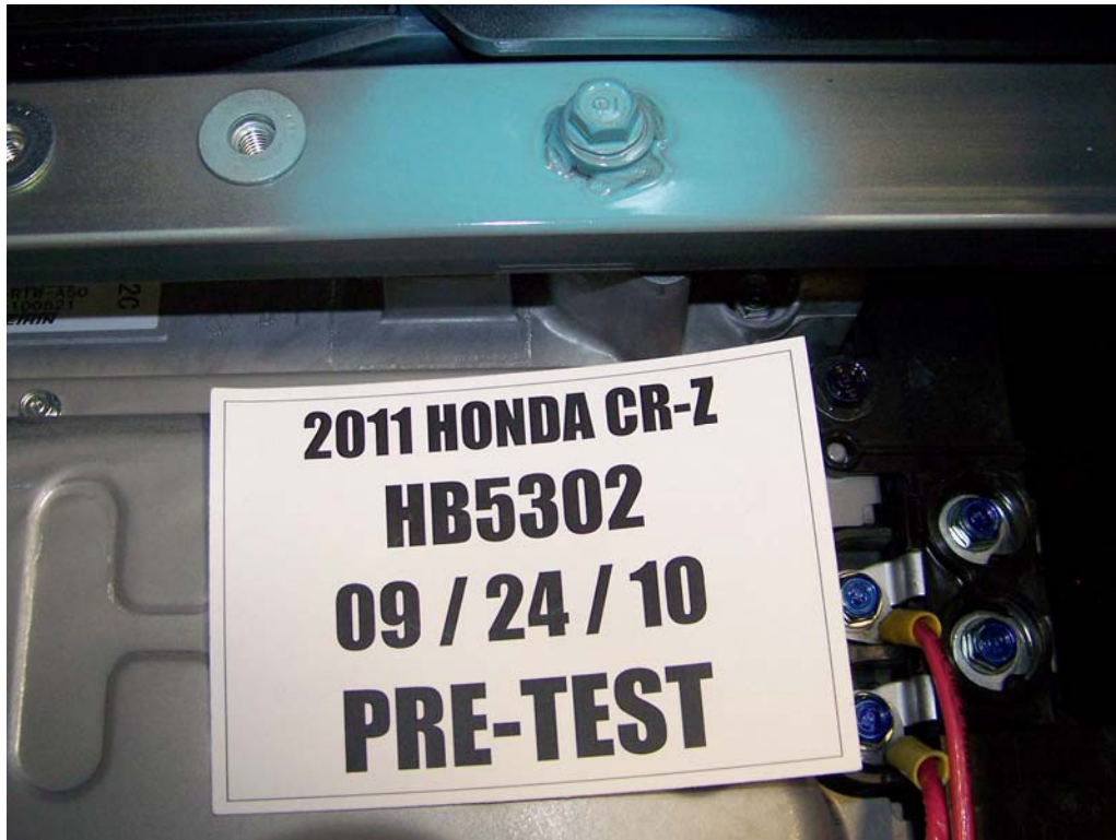
FIGURE 103. Pre-Test Battery Mounting Hardware
