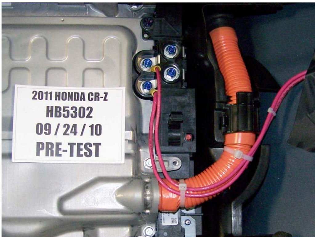
FIGURE 76. Pre-Test Electrical Propulsion Components
