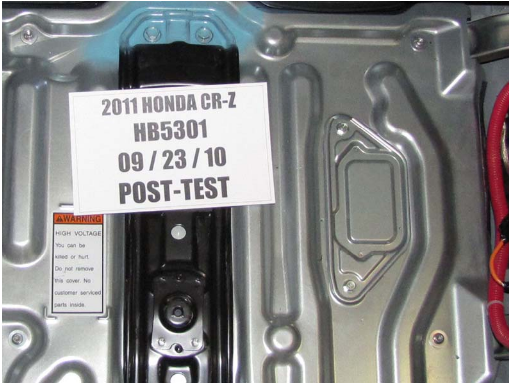
FIGURE 114. Post-Test Propulsion Battery Disconnect
