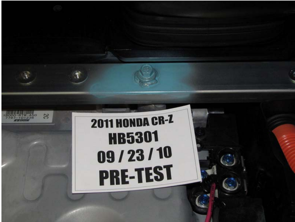
FIGURE 134. Pre-Test Battery Mounting Hardware
