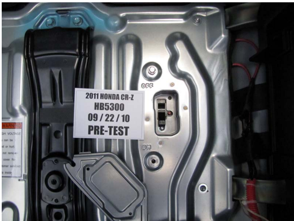
FIGURE 82. Pre-Test Propulsion Battery Disconnect
