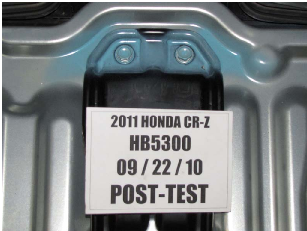
FIGURE 86. Post-Test Battery Mounting Hardware
