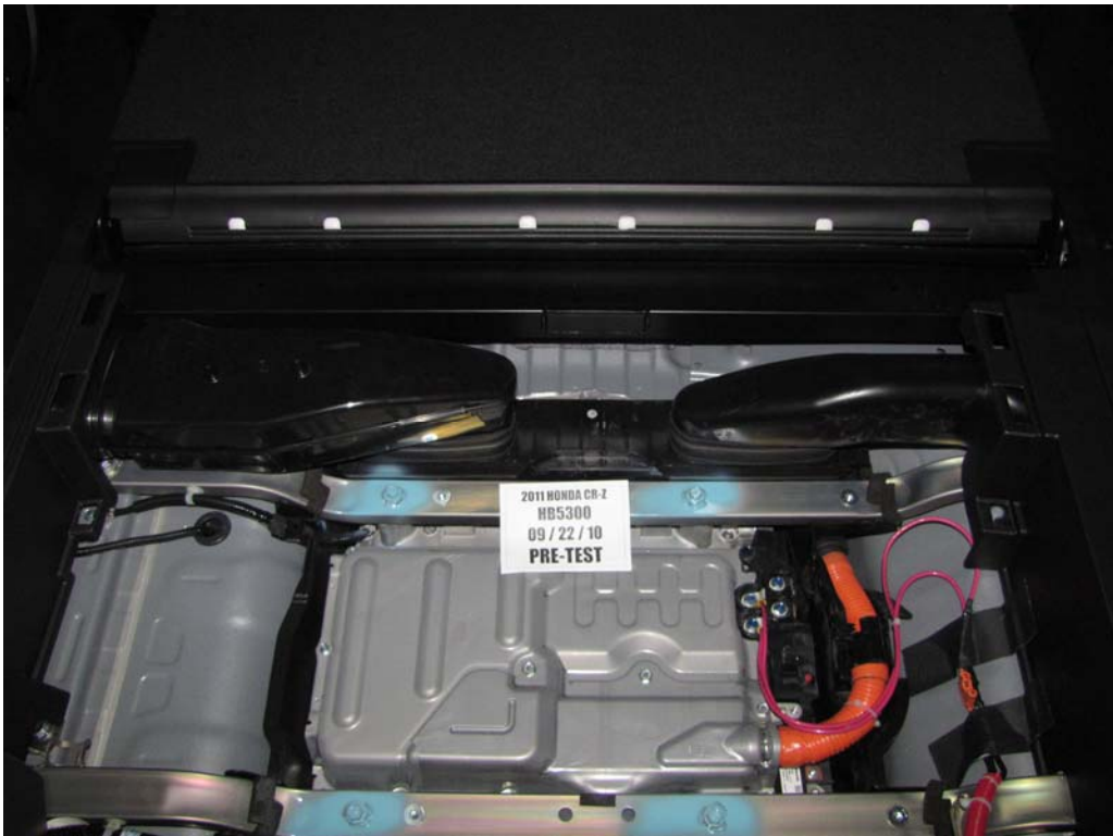
FIGURE 78. Pre-Test Battery Compartment
