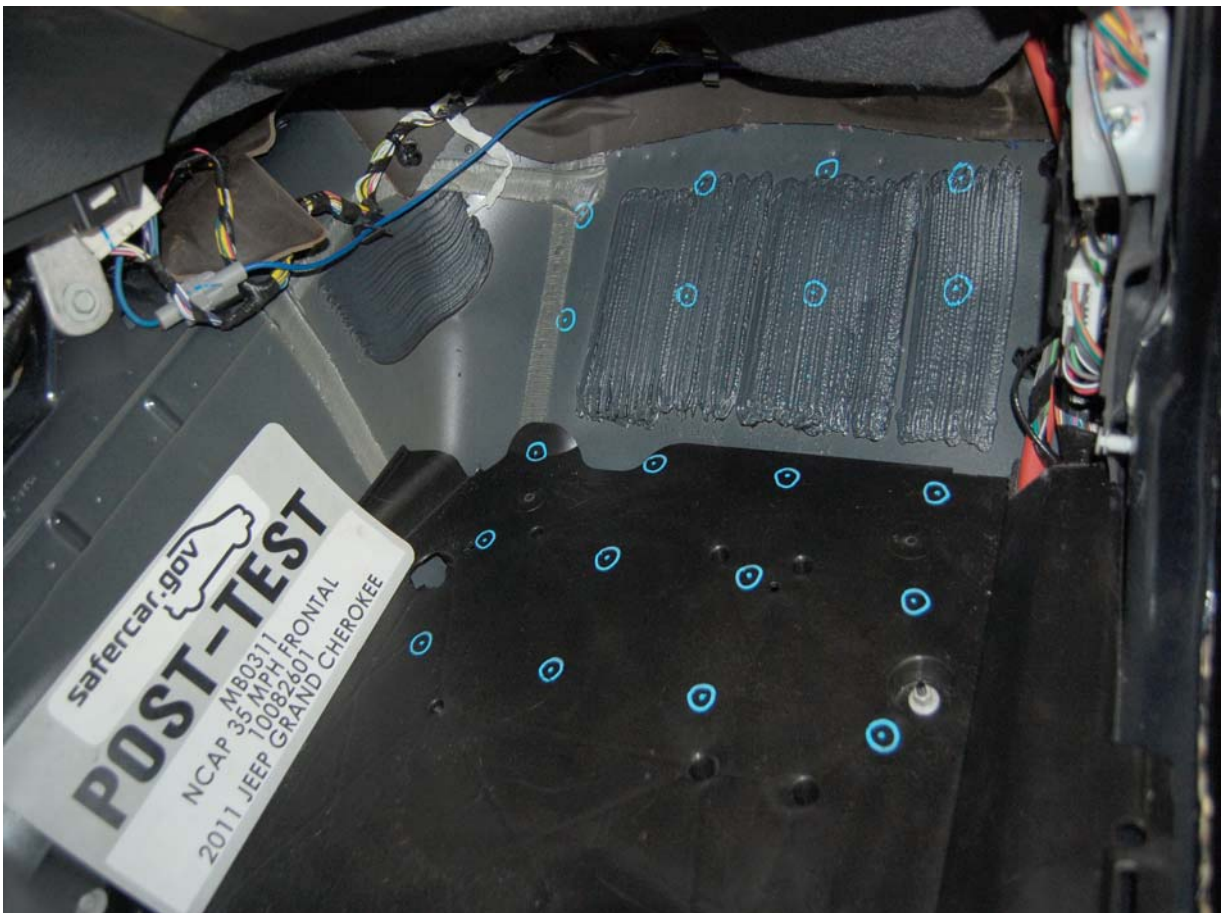
Post-Test Passenger's Side Floorpan
