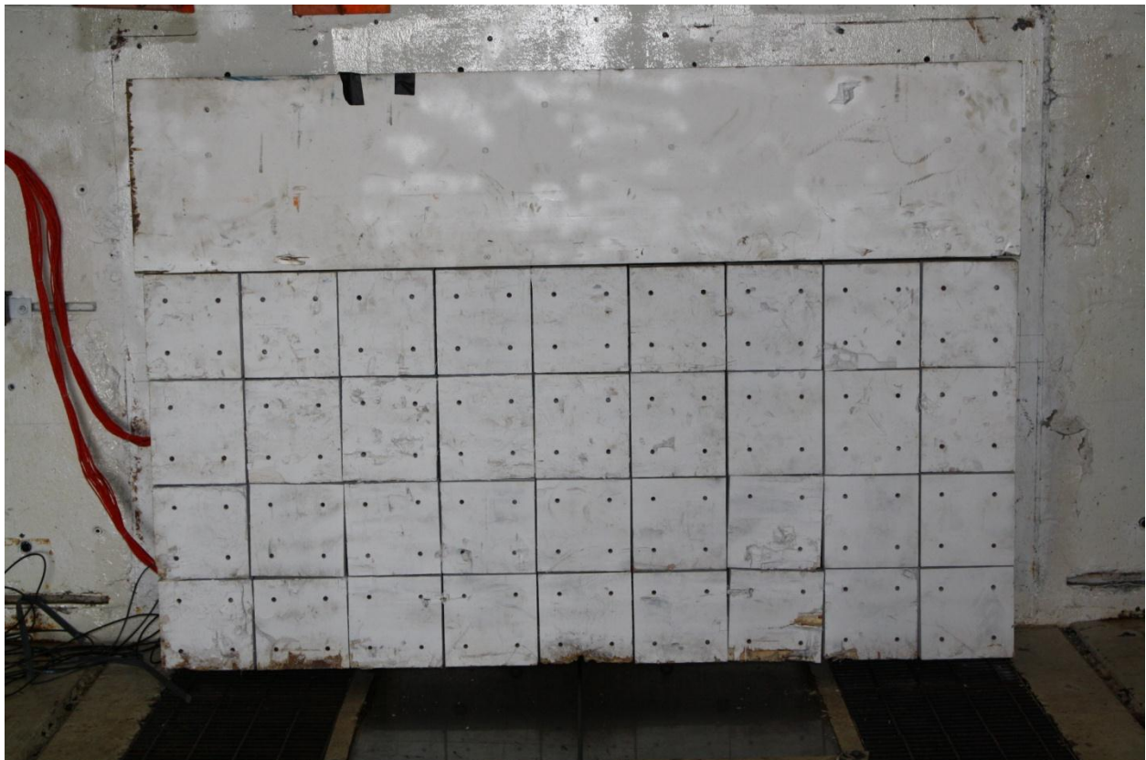
Figure A-2: Load Cell Wall
