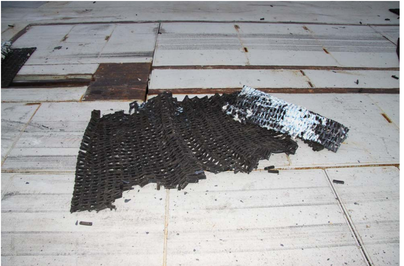
Figure A-68 Post-Test Mat Displacement – View 5
