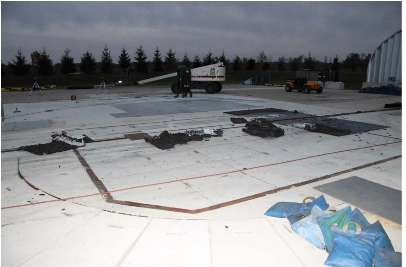
Figure A-66 Post-Test Mat Displacement – View 3
