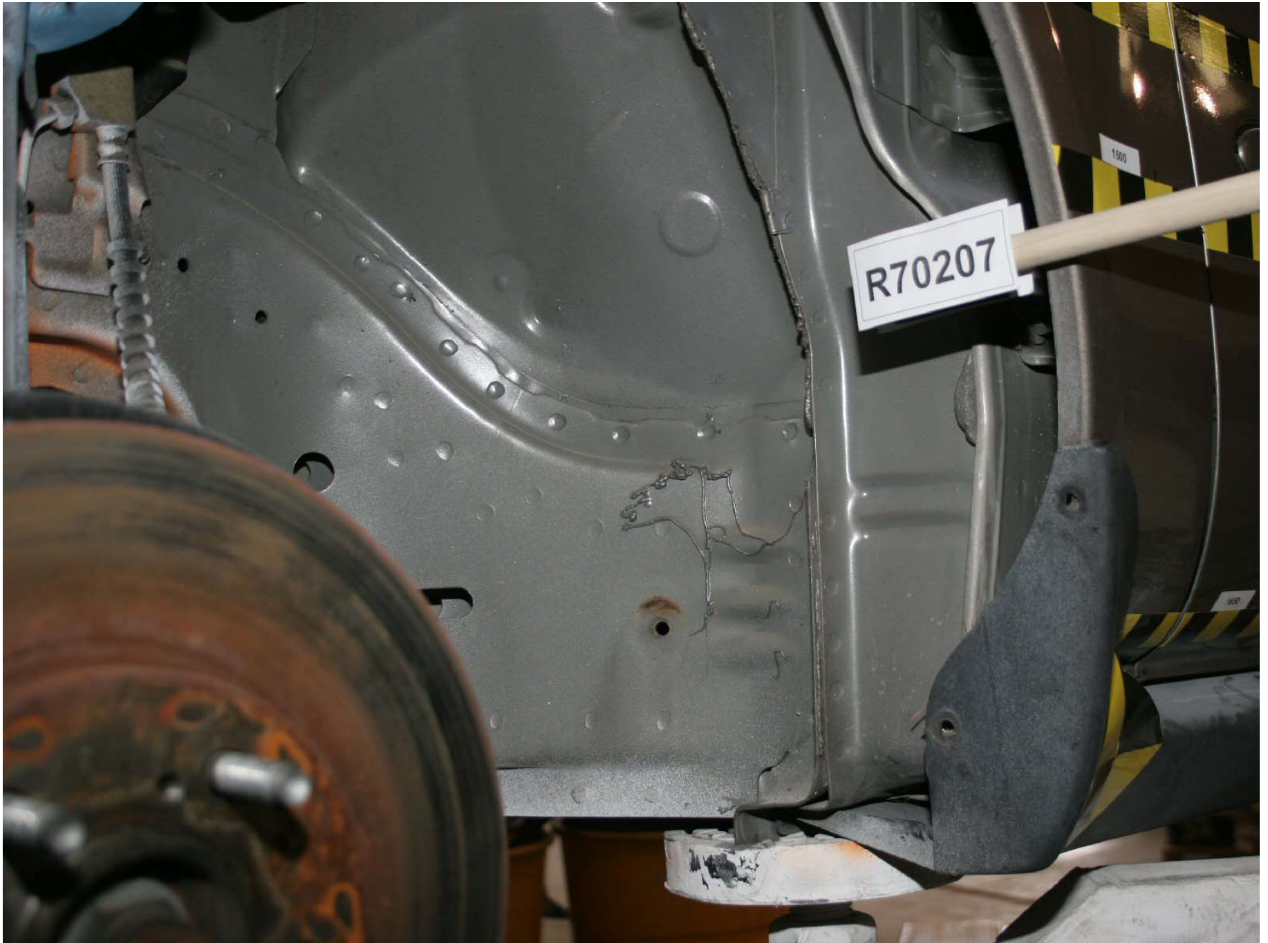
Figure A-157: Test Vehicle Pre-Test Left Side Frame to A-Pillar Joint
