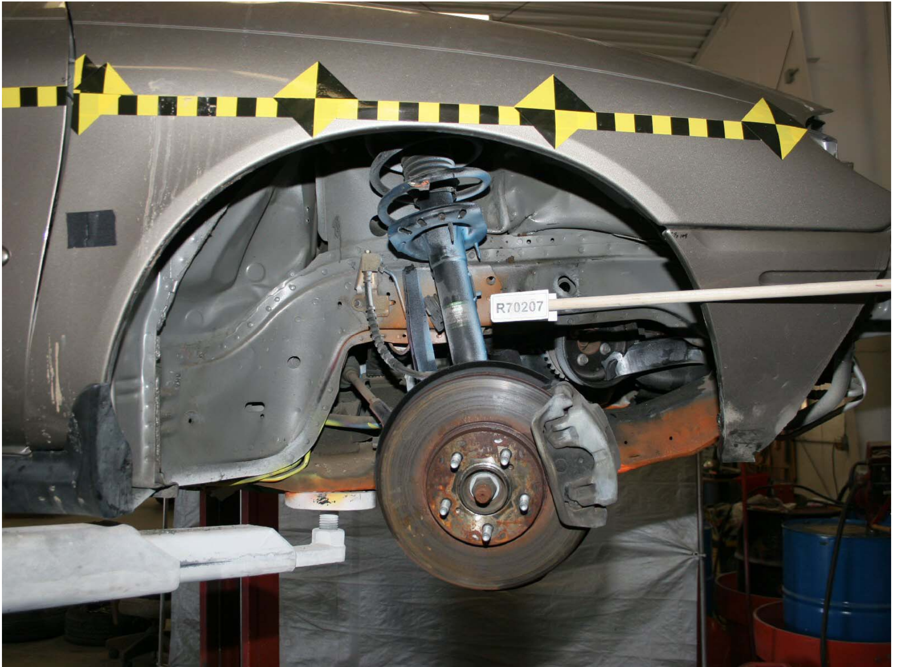
Figure A-174: Test Vehicle Post-Test Right Front Wheel Well (Tire Off), Inner Fender Removed
