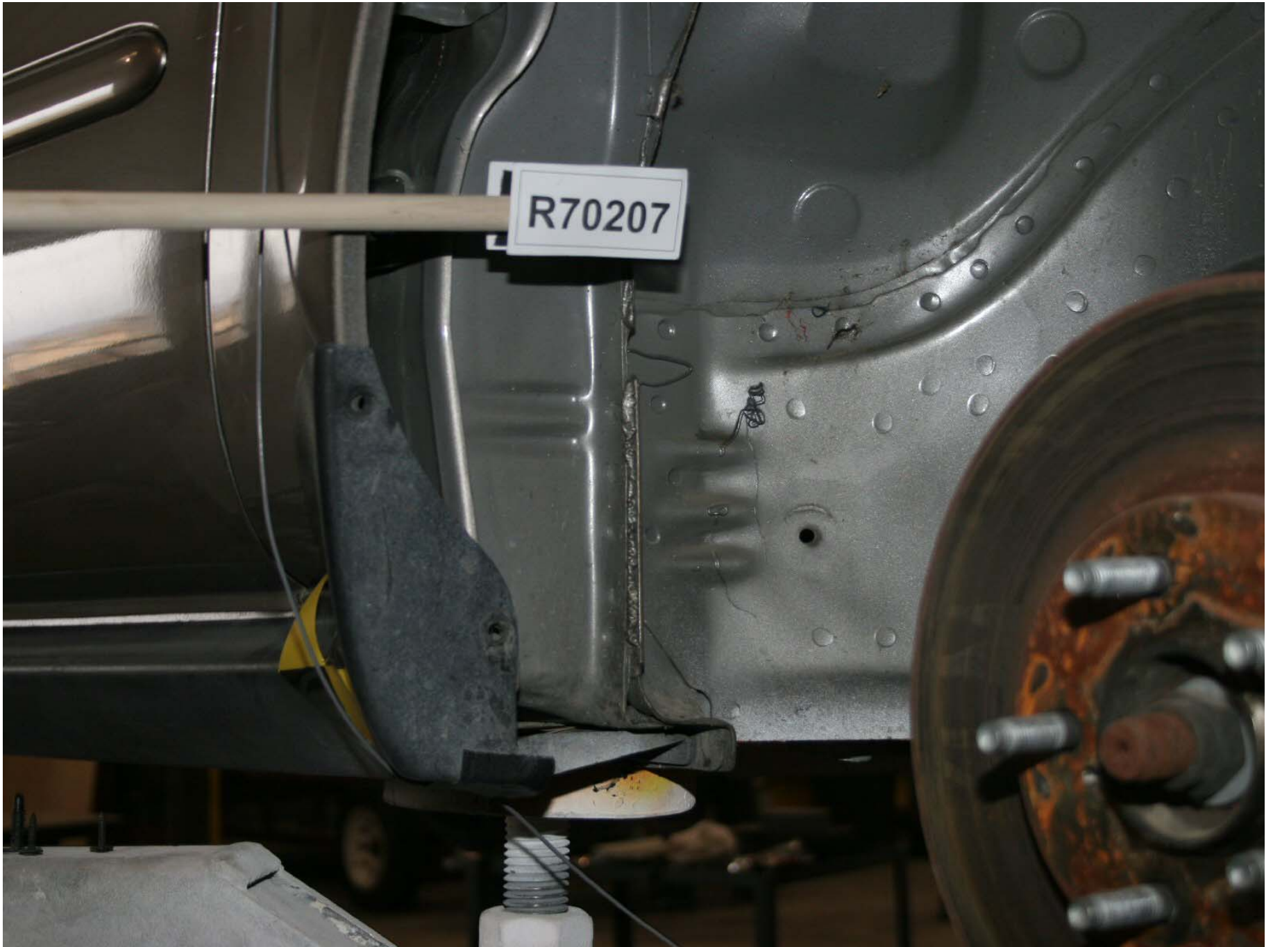
Figure A-193: Test Vehicle Pre-Test Right Side Upper Sway Bar Attachment Point
