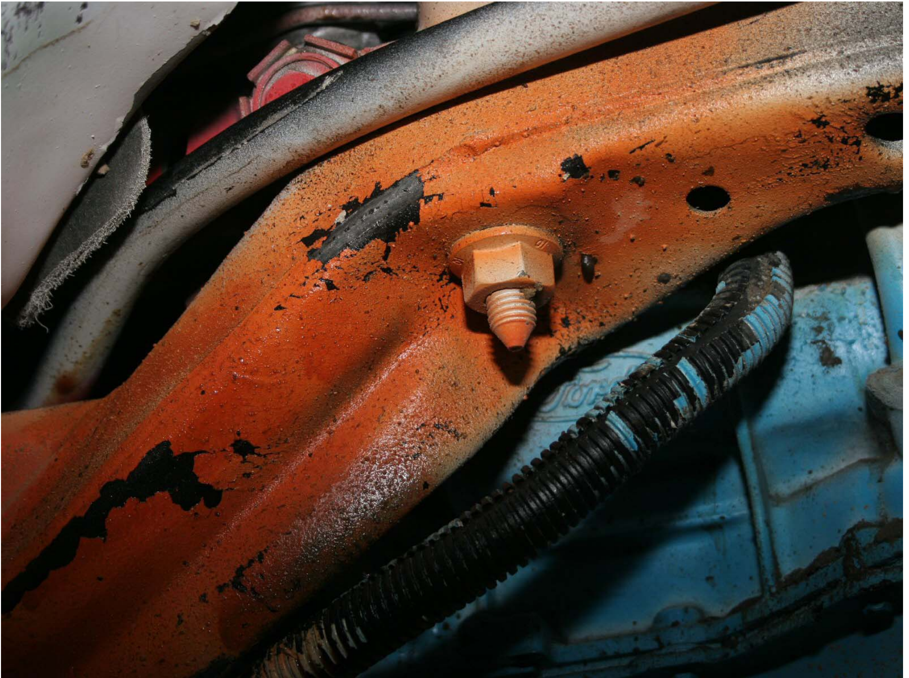
Figure A-213: Test Vehicle Post-Test Steering Rack Left Side Mounting Bolt
