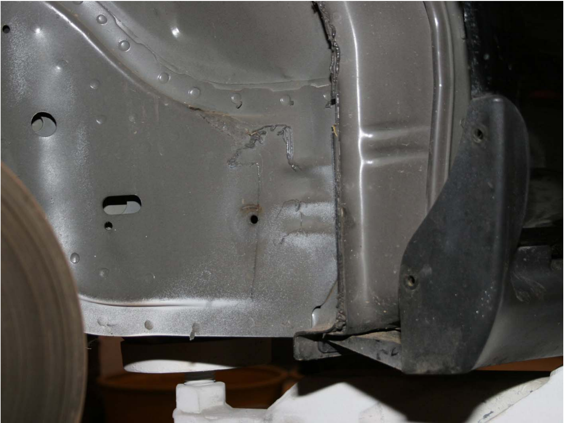
Figure A-156: Test Vehicle Pre-Test Left Side Frame to A-Pillar Joint
