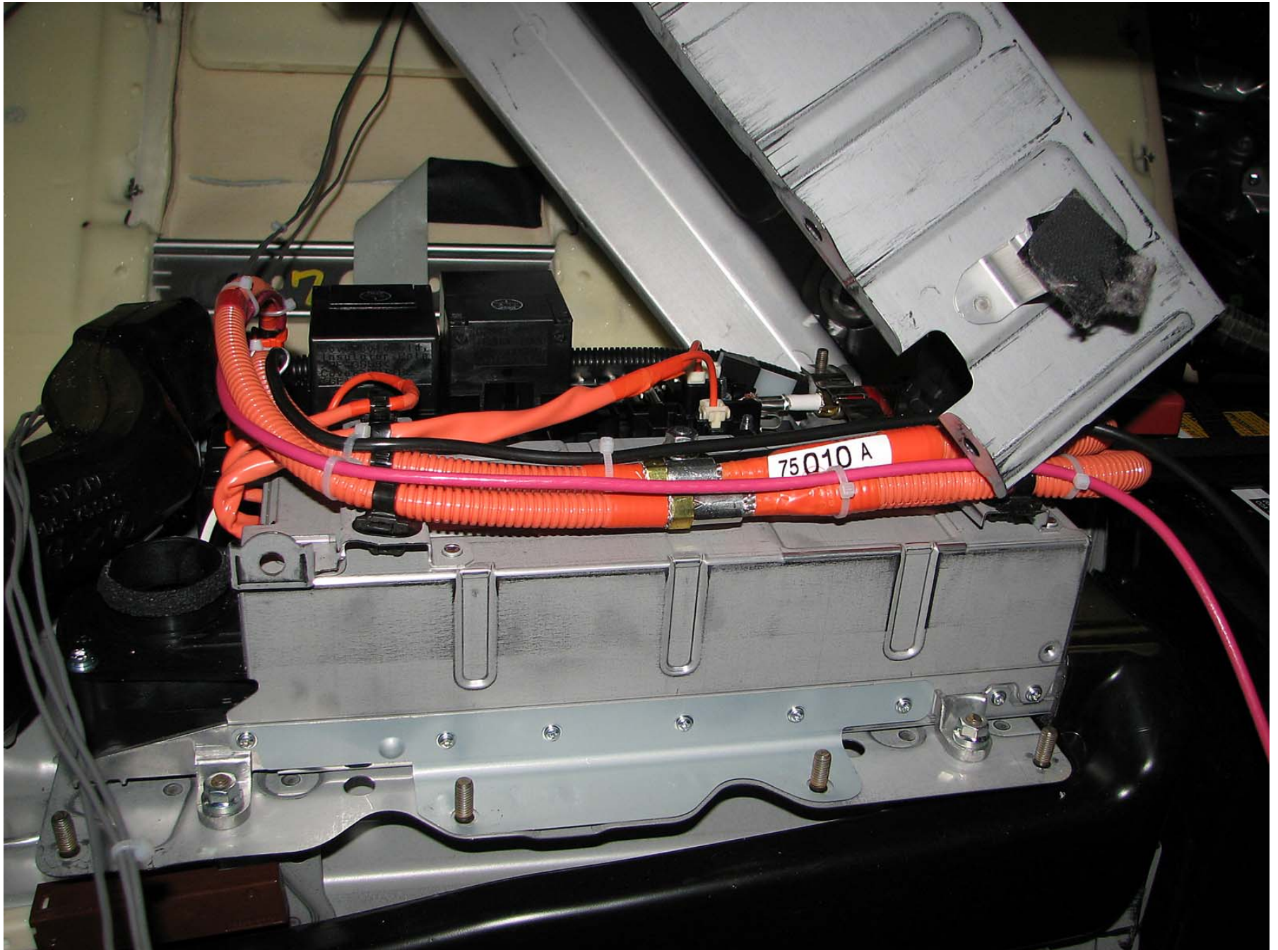
Figure A-67: Pre-Test View of Battery Compartment
