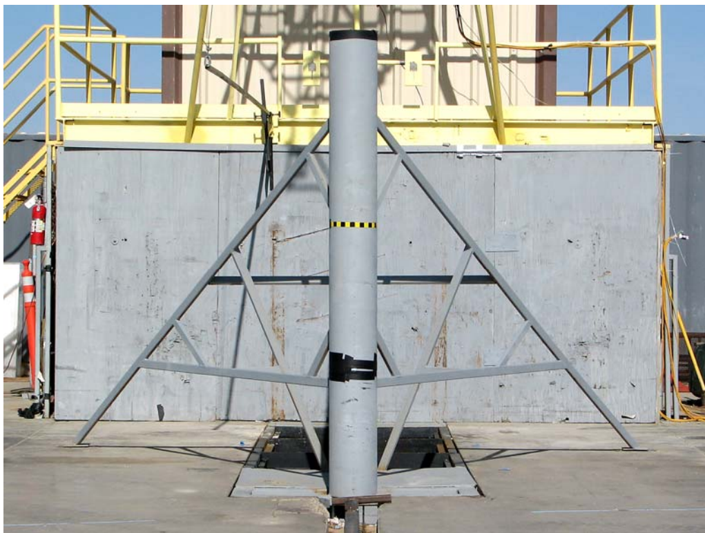
FIGURE 42. Pre-Test Pole Barrier Front View
