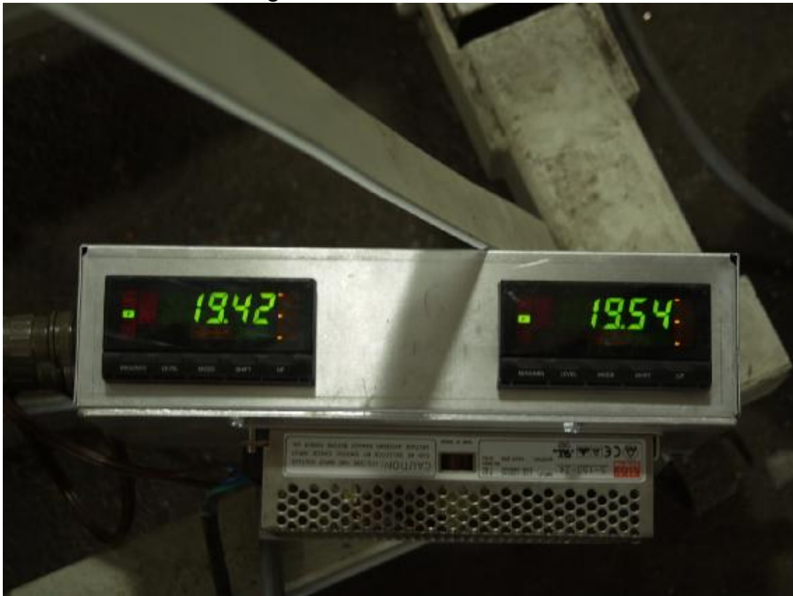
Figure A-46: Post-Test Primary and Redundant Speed Trap Read-
