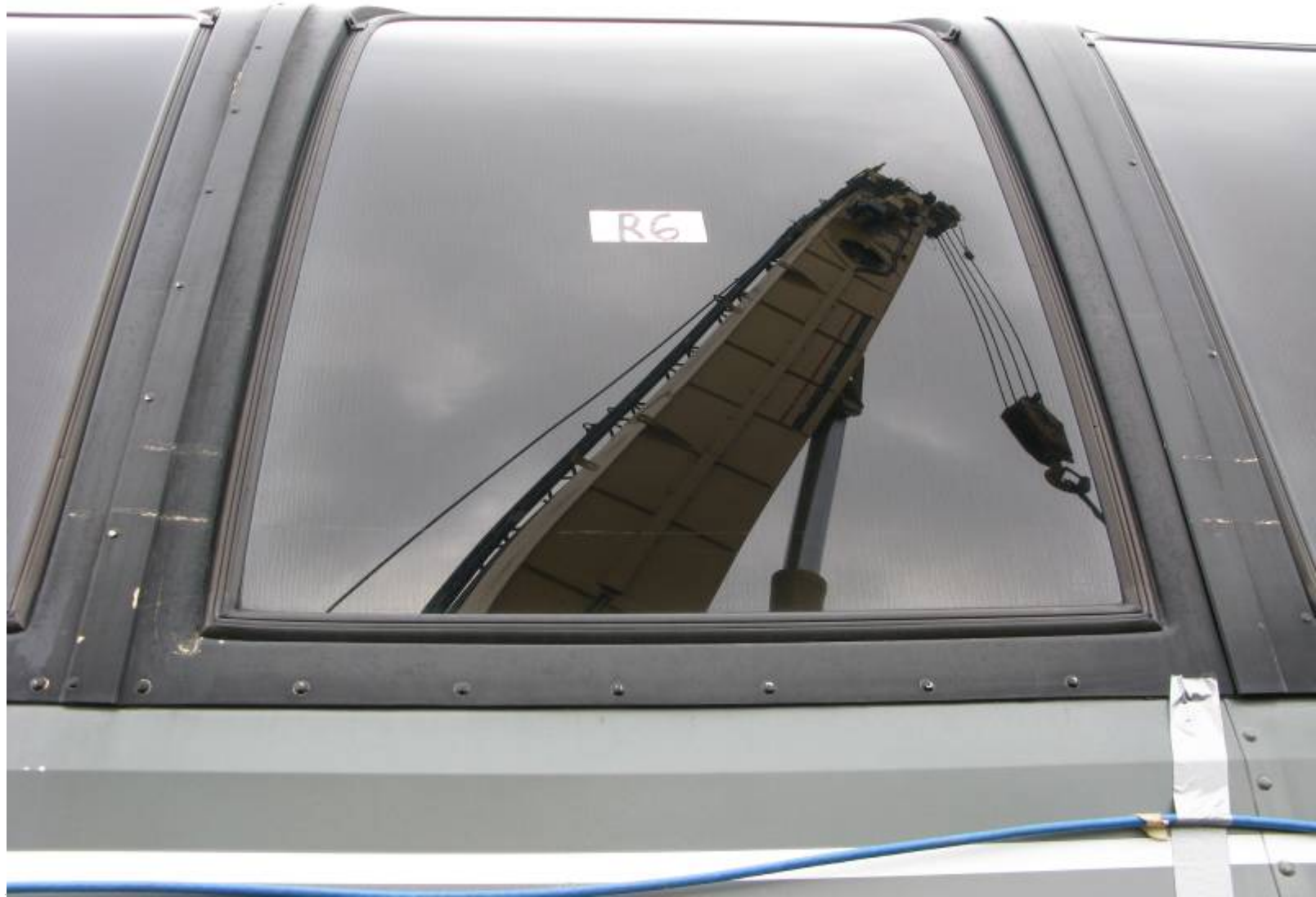
Pre-Test Right Side Window 6 Exterior View
