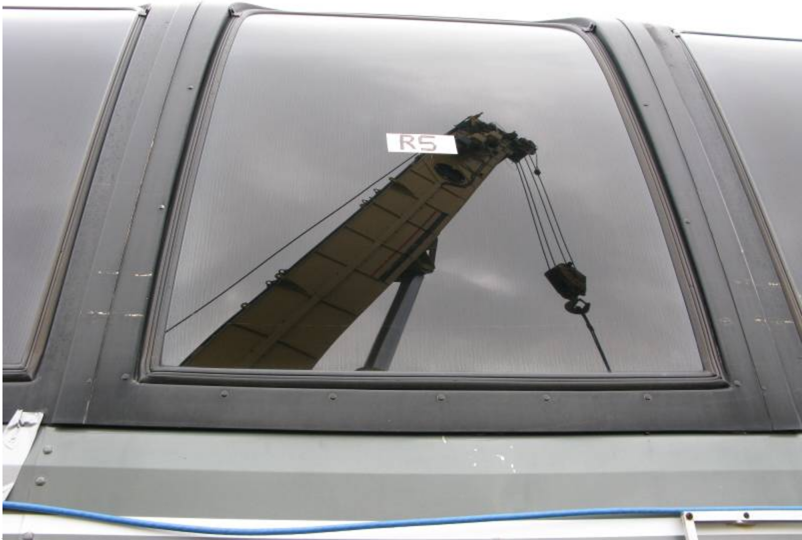
Pre-Test Right Side Window 5 Exterior View
