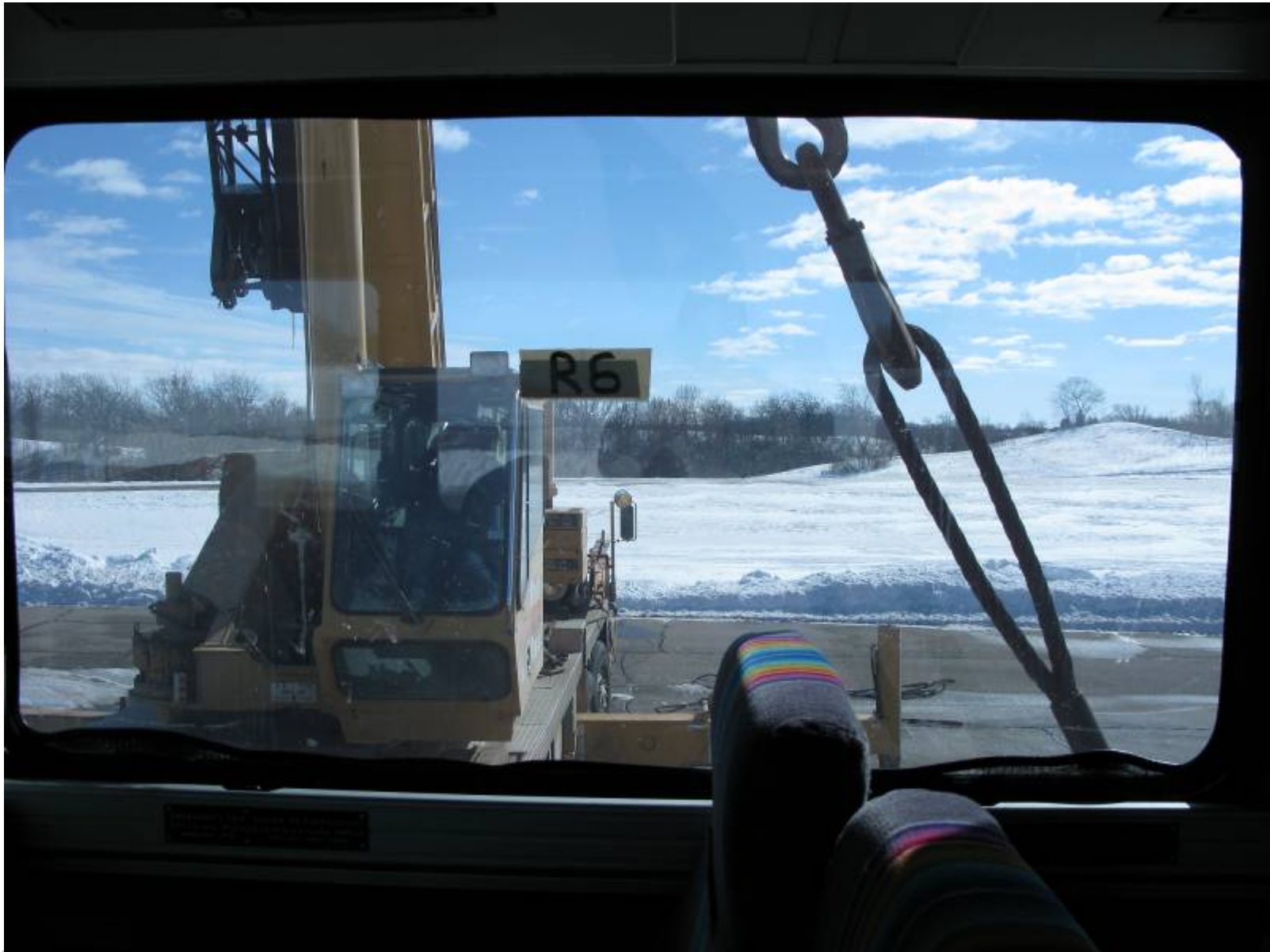
Pre-Test Right Side Window 6 Interior View
