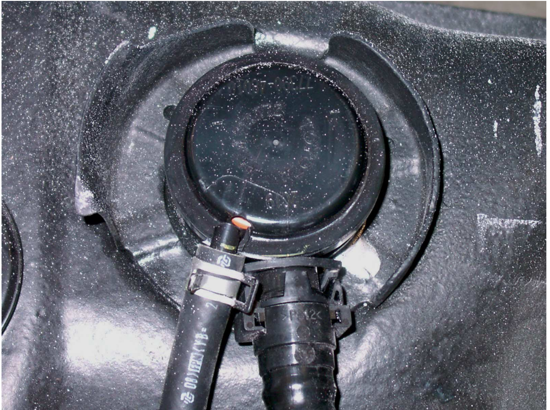
Figure A-61: Damage to Fuel System, Post-test
