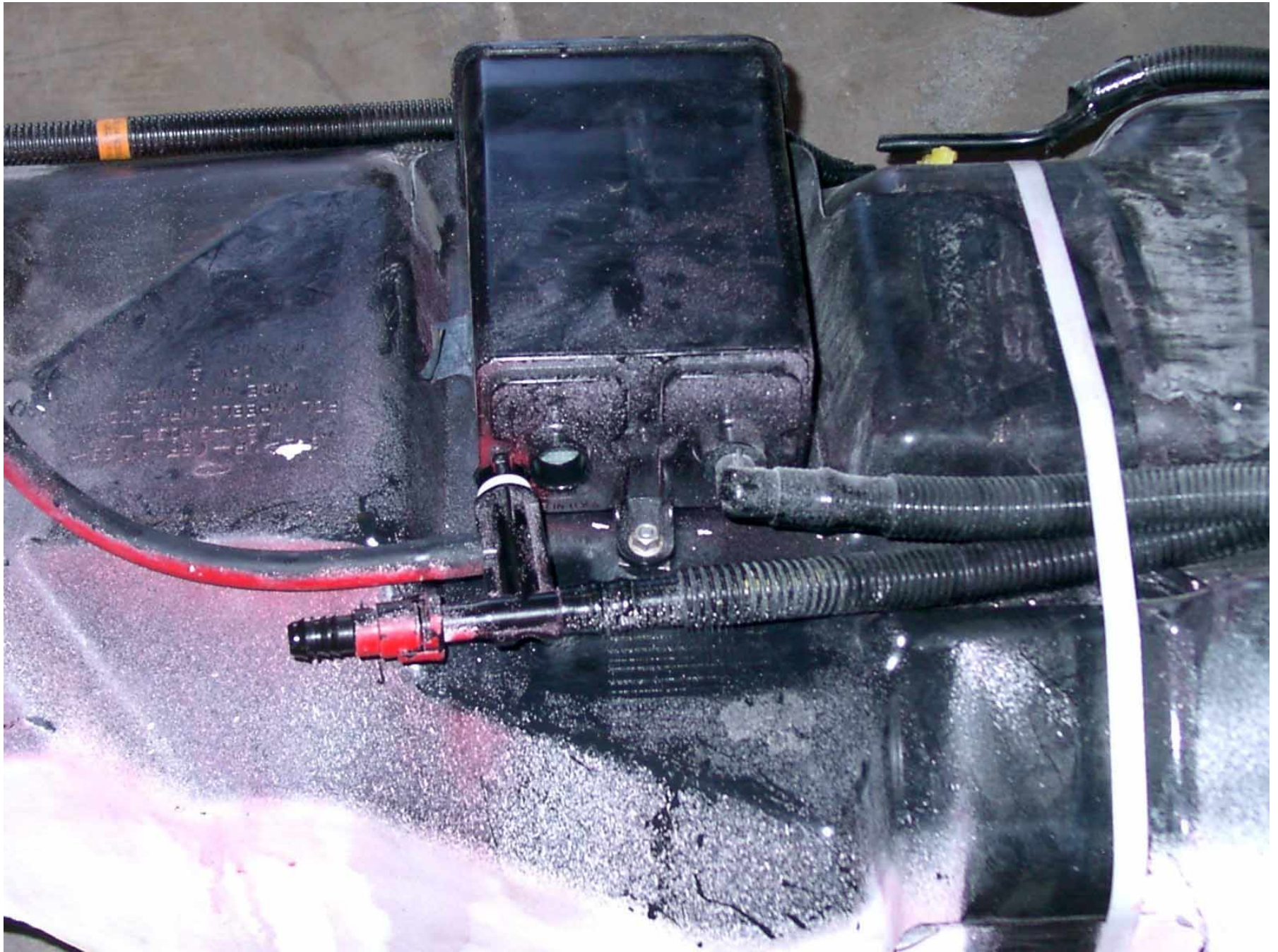
Figure A-61: Fuel System Spillage Detail
