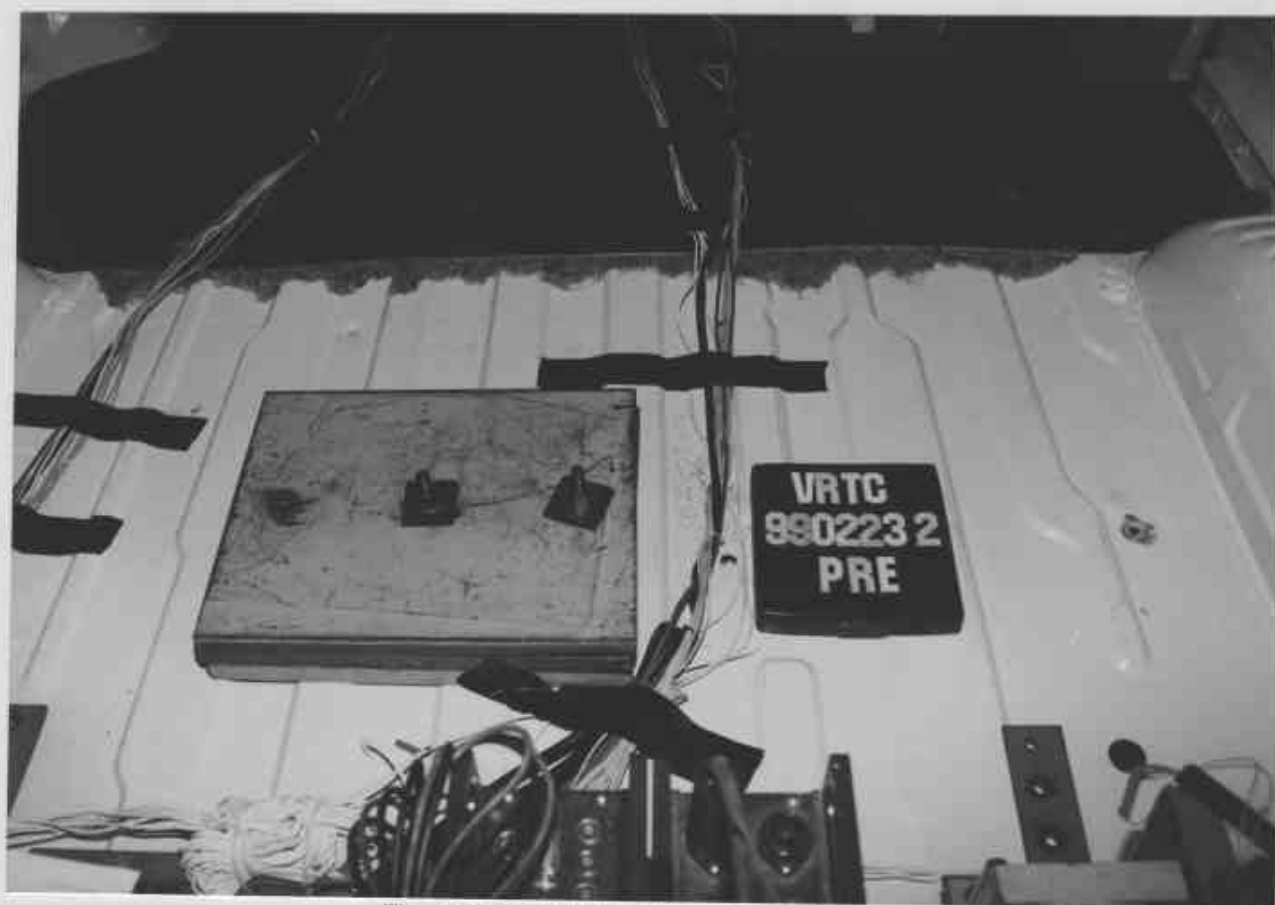
Figure A-58 Pre-Test Ballast Location View
