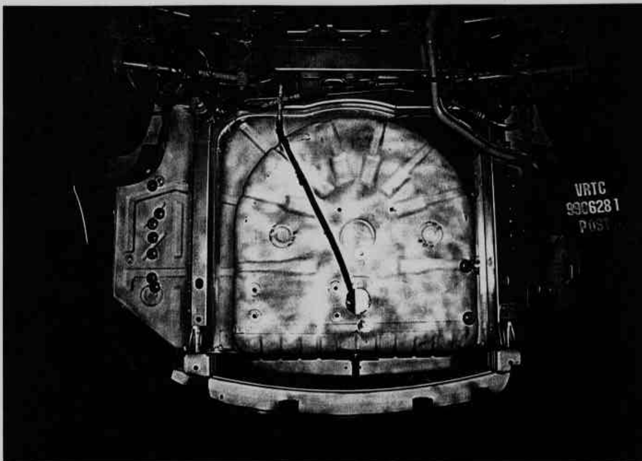
Figure A-26 Post-Test Underbody - View 5
