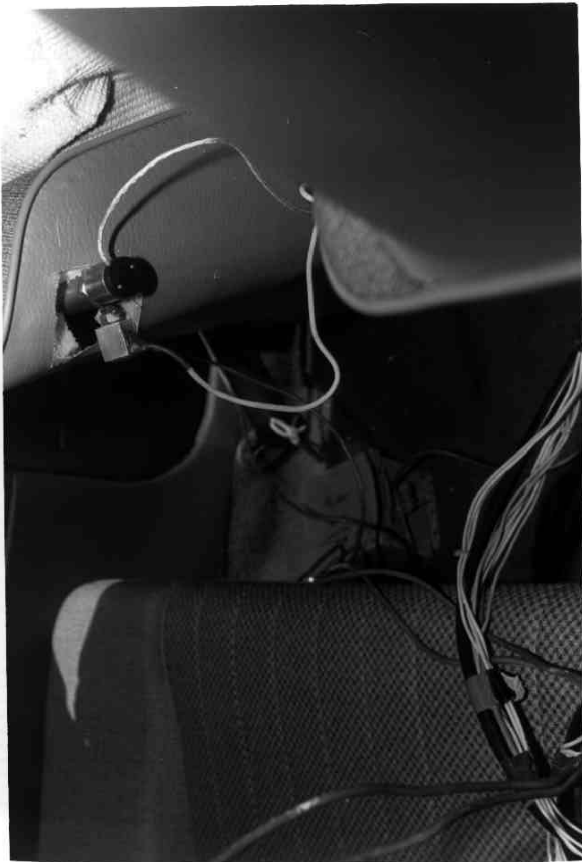
FIGURE 5-17 SEAT FRAME MOUNTED ACCELEROMETERS AND MHD SENSOR
