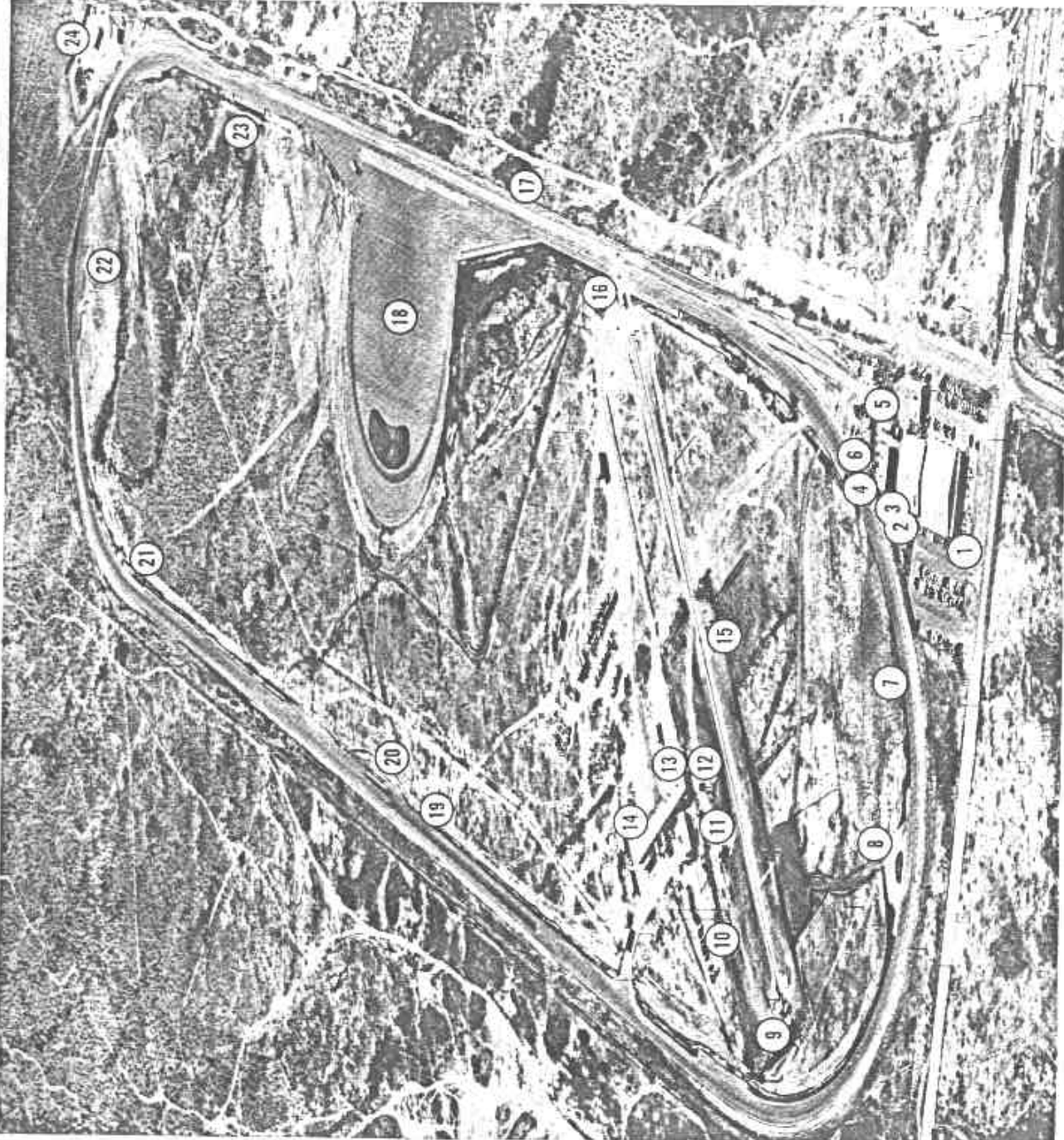
Figure A-1. The Dynamic Science, Inc. Phoenix Facility.
